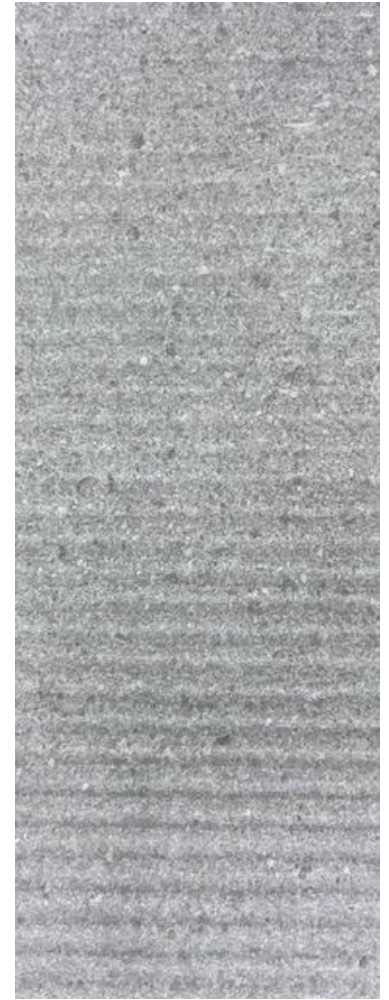
TILE ON TUB WALL
