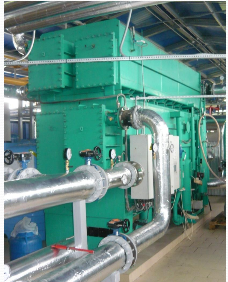
Absorption lithium bromide refrigerating machine (ABHM)
