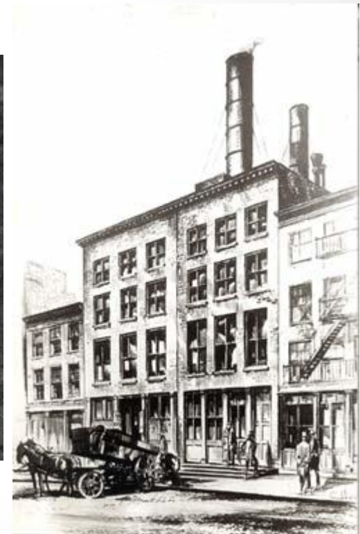
A sketch of the exterior of the Pearl Street station, New York, 1882
