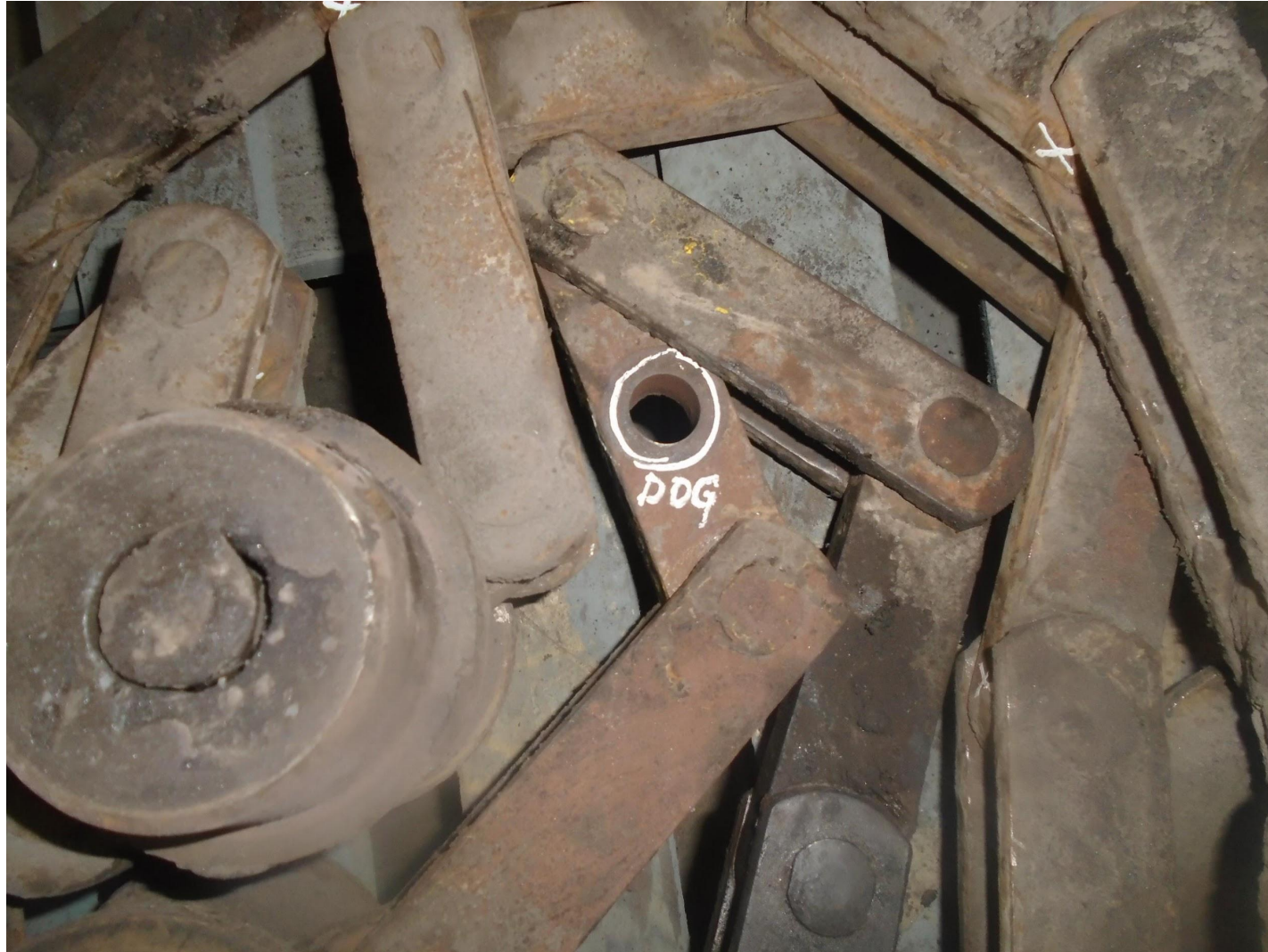
Dog mounting shaft hole badly worn out
