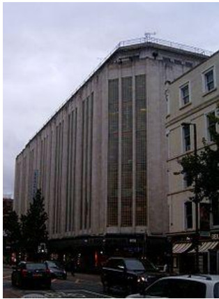
Kendals department store in Manchester, England.
