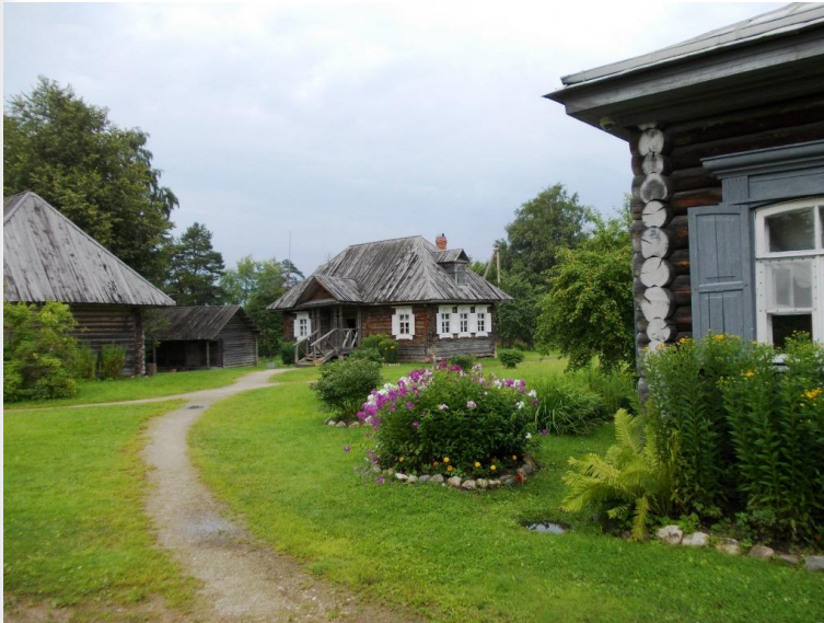
The kitchen outbuilding
