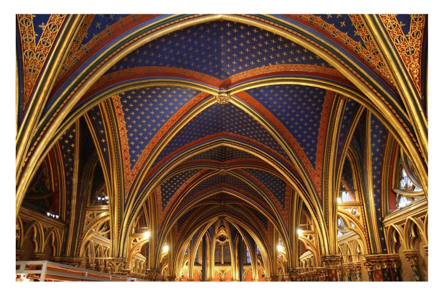
IN ARCHITECTURE, A VAULT IS A SELF-SUPPORTING ARCHED FORM, USUALLY OF STONE OR BRICK, SERVING TO COVER A SPACE WITH A CEILING OR ROOF.
