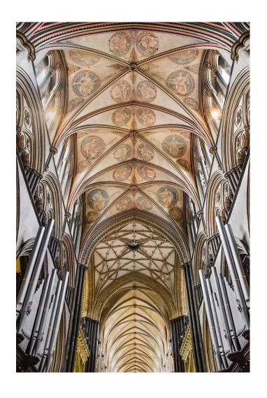
When two semicircular barrel vaults of the same diameter cross one another their intersection (a true ellipse) is known as a groin vault
