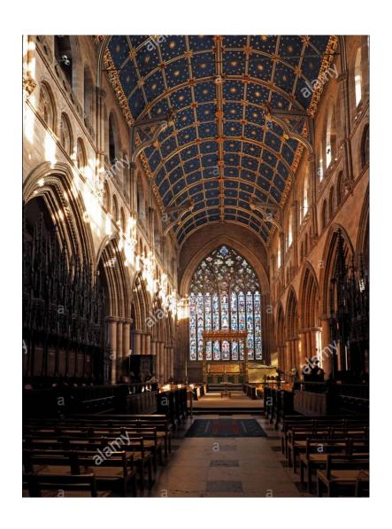
A barrel vault is the simplest form of a vault and resembles a barrel or tunnel cut lengthwise in half. The effect is that of a structure composed of continuous semicircular or pointed sections.
