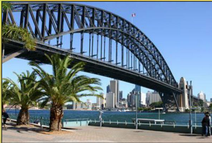
The Harbour Bridge
