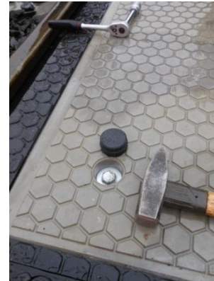
Placing concrete elements in rubber
