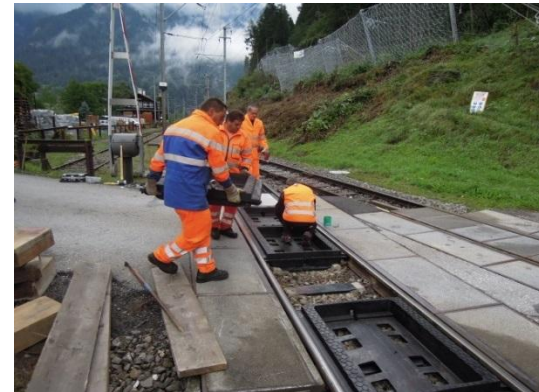
Installation of rubber elements
