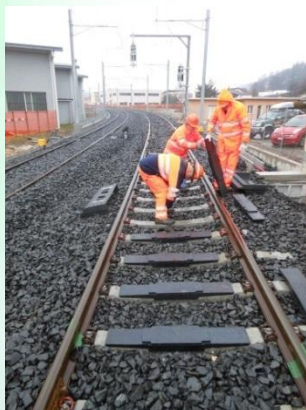
Cleaning of the track and installation of supports
