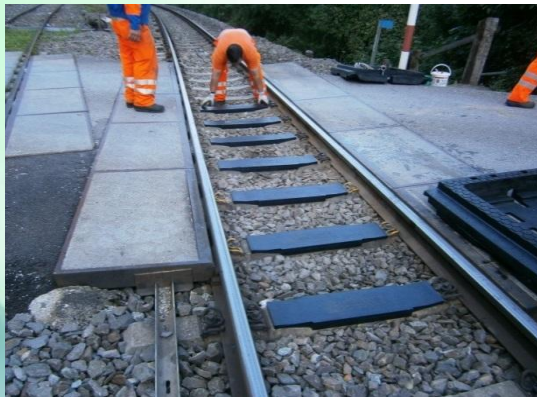
Cleaning of the track and laying of supports
