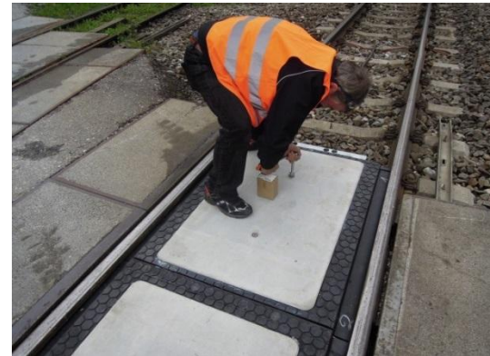
Place concrete elements to rubber
