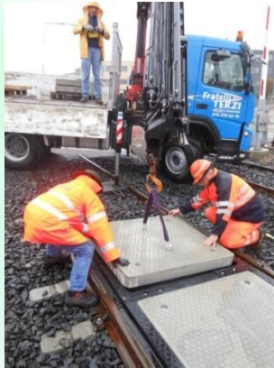
Placing concrete elements in rubber
