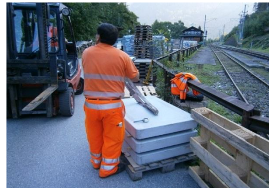
Moving concrete using a power-driven wagon
