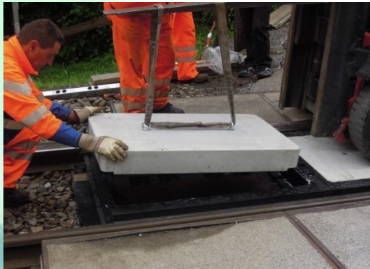
Place concrete elements in rubber
