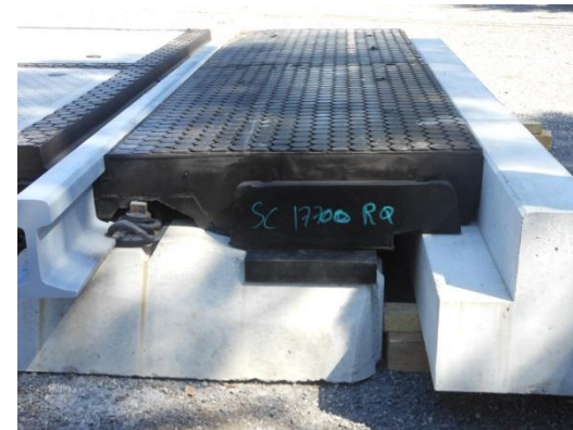
Installing side elements
