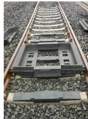
Laying of rubber elements (shoe and spacer)
