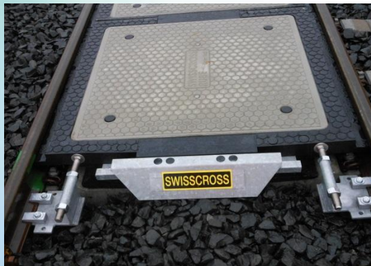
Installing of accessories
