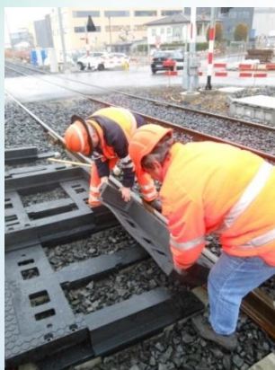
Laying of rubber elements (shoe and spacer)
