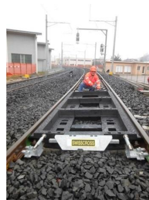
Laying of rubber elements (shoe and spacer)
