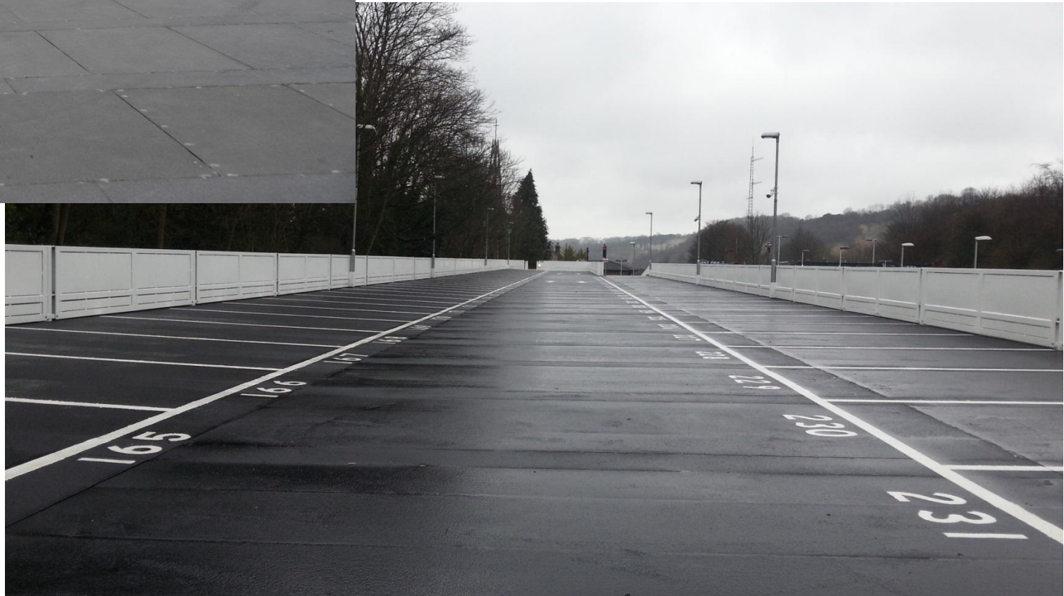
Gen 4 Panels Sealed infill panels water drains to slot channel then to std ali gutter
