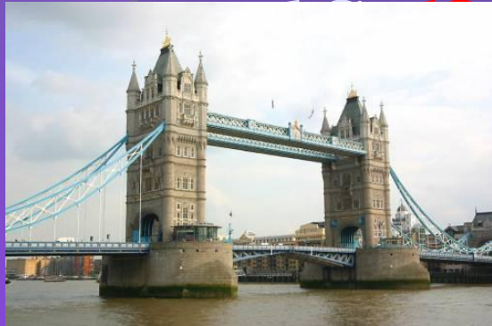
a) Tower Bridge
