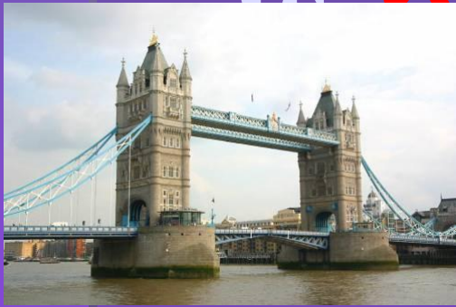
a) Tower Bridge
