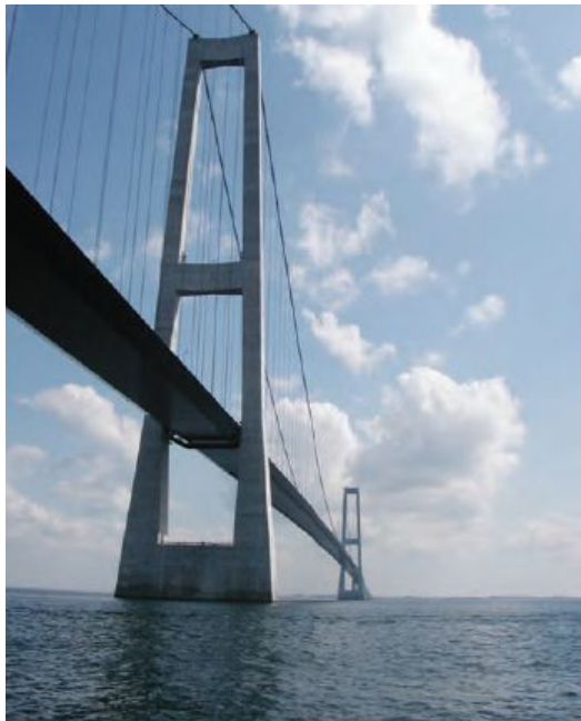
▲ Figure 7.48 The Great Belt East Bridge of Denmark is 6.8 km long and is constructed with a smooth underside. This allows air to flow by without inducing a resonant frequency.
