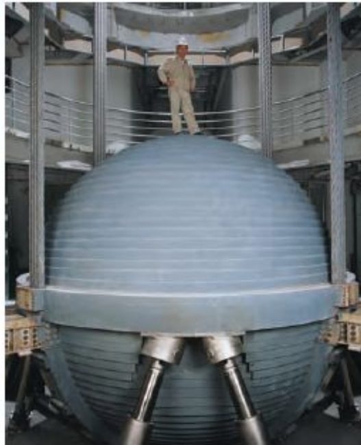
▲ Figure 7.49 The Taipei 101 building in Taiwan was completed in 2004 and stands 101 stories high. The inset shows a tuned mass damper in the building designed by Motioneering Inc. of Guelph, Ontario. It has a huge mass and vibrates opposite to the direction of the building, cancelling much of the amplitude of the resonant vibration.
