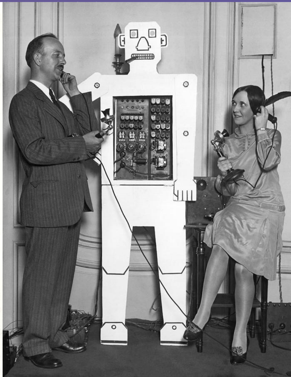
Fig. 476 The Televox made by the engineer Wensley, Pittsburgh.
