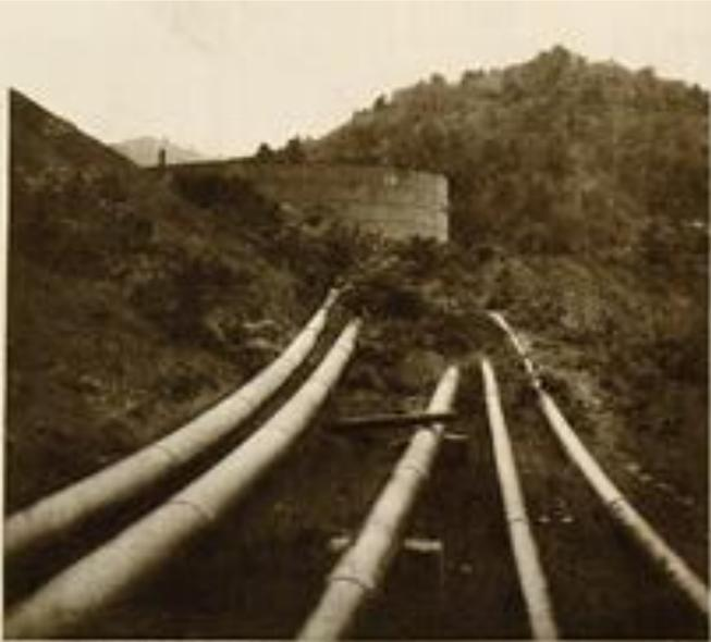
Fig. 1. Pipes for the transport of water from the reservoir to the power station.
