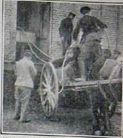
**New travelling boiler now part of the German Red Cross equipment. By an ingenious process water is drawn from wayside streams and ponds and filtered simultaneously.**
