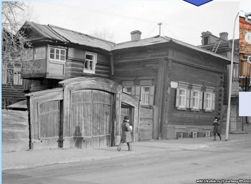
The Shubin's mansion (1781) – Lapina st.
