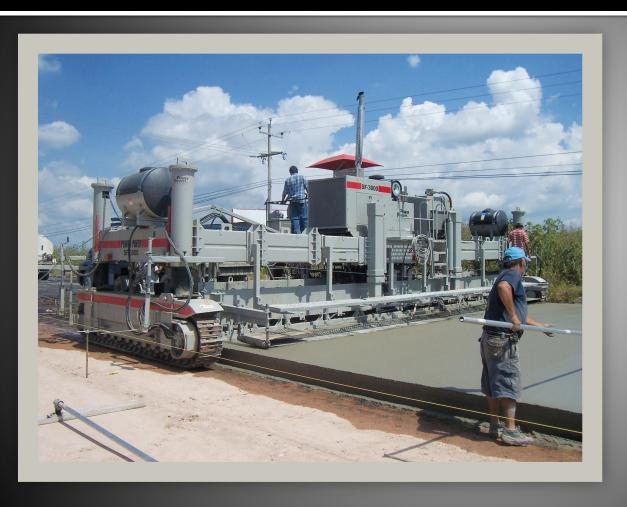
The concrete is supplied by truck mixers or is dumped between the forms and spread with a crane
