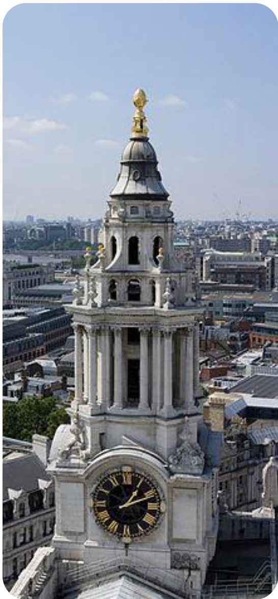
South west tower of St. Paul's Cathedral.
