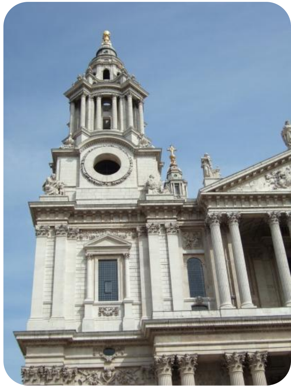
West side of the north tower of St Paul's Cathedral.
