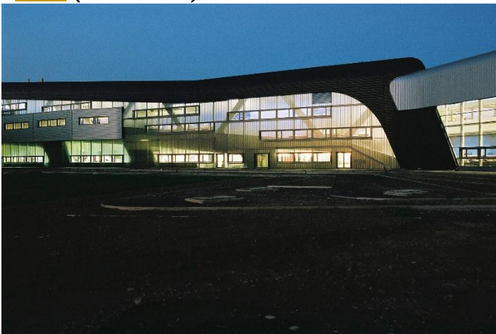
Administration building of BMW Factory in Leipzig , Germany (2001–2005)
