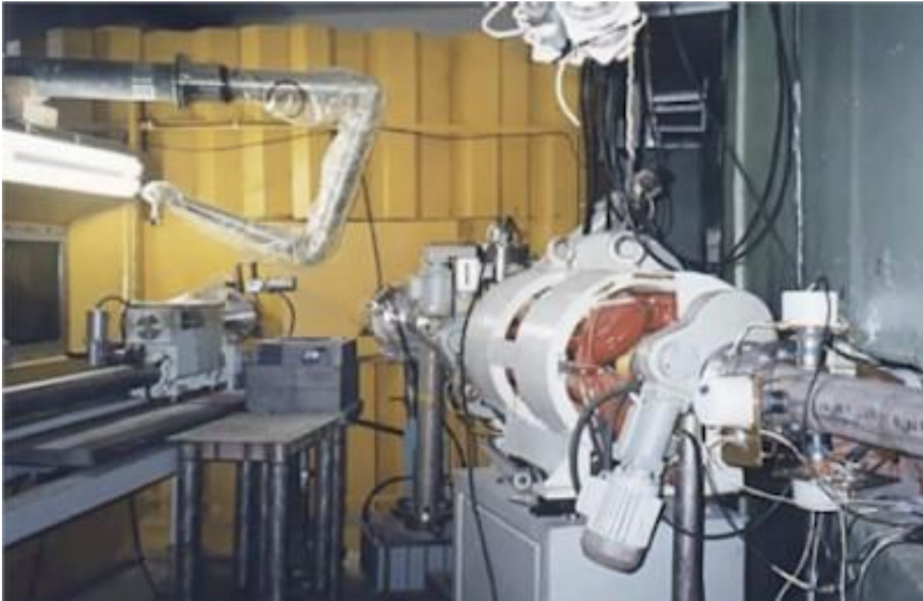
The Central part of the radionuclide production facility at a linear proton accelerator with an energy of up to 160 MeV
