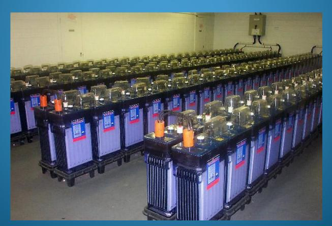
**Accumulator** - a set of positive and negative electrodes disposed in the reservoir with electrolyte and intended to convert accumulated chemical energy into electrical energy.
