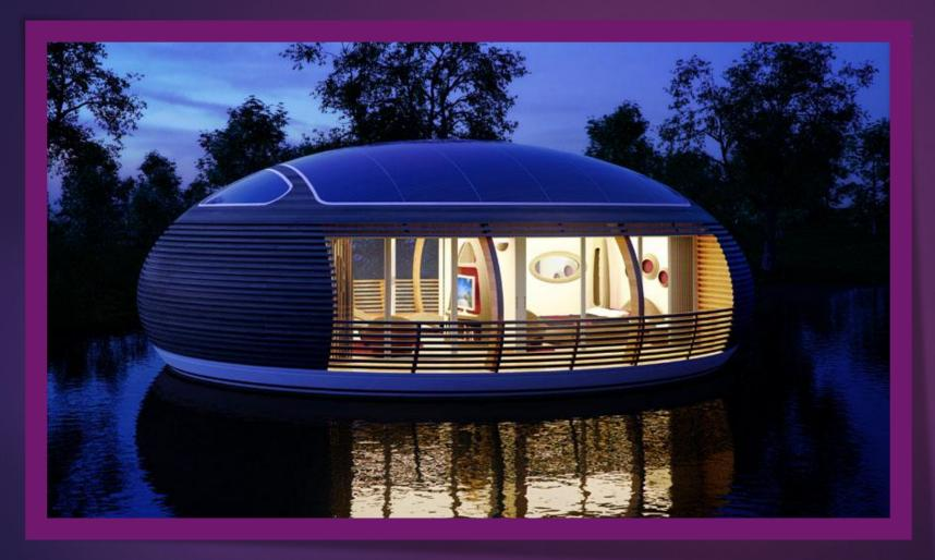
On the rounded wooden roof photovoltaic panels are installed. The total area of panels is 60 square meters, which is able to develop up to 4 kWp of electricity per hour. Large windows and balconies around the house will allow guests enjoy beautiful peaceful views of water.
