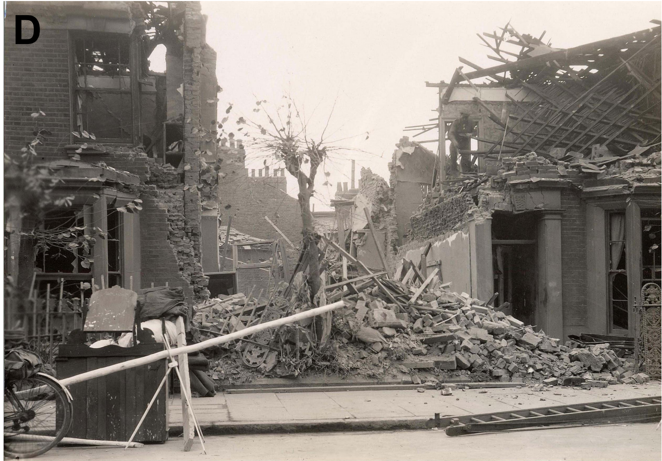
Bomb damage to 30 Gayhurst Road, Hackney, following an attack by the German Air Force with high explosive bombs on 15/16 October 1940.
