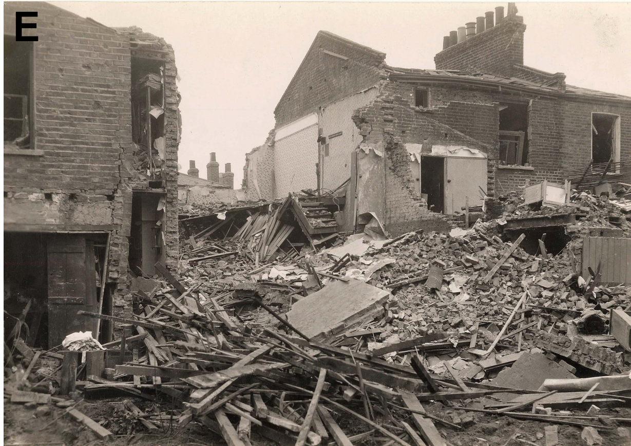
Bomb damage to 60-64 Lansdowne Drive, following an attack by the German Air Force with high explosive bombs on 15/16 October 1940.
