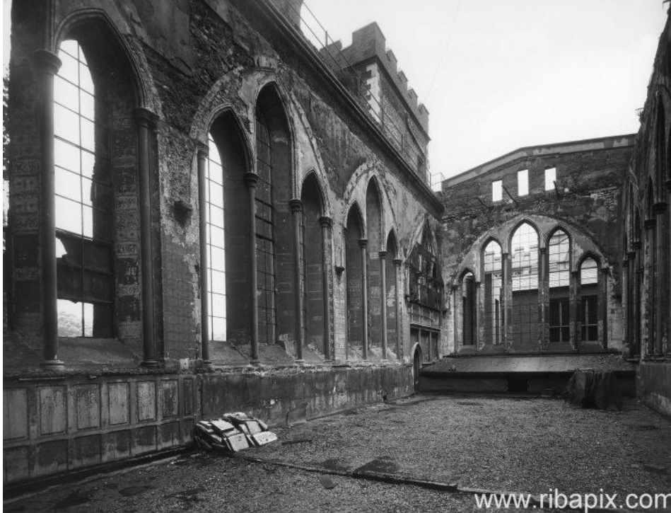
Lambeth Palace, London: the remains of the chapel after bomb damage, 1950's
