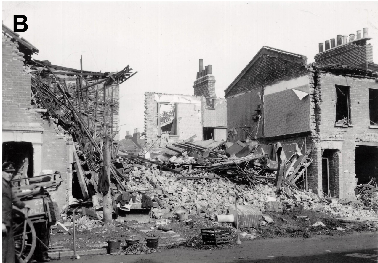
Bomb damage to 117-121 Mapledene Road, Hackney, following an attack by the German Air Force with high explosive bombs on 09/10 October 1940.
