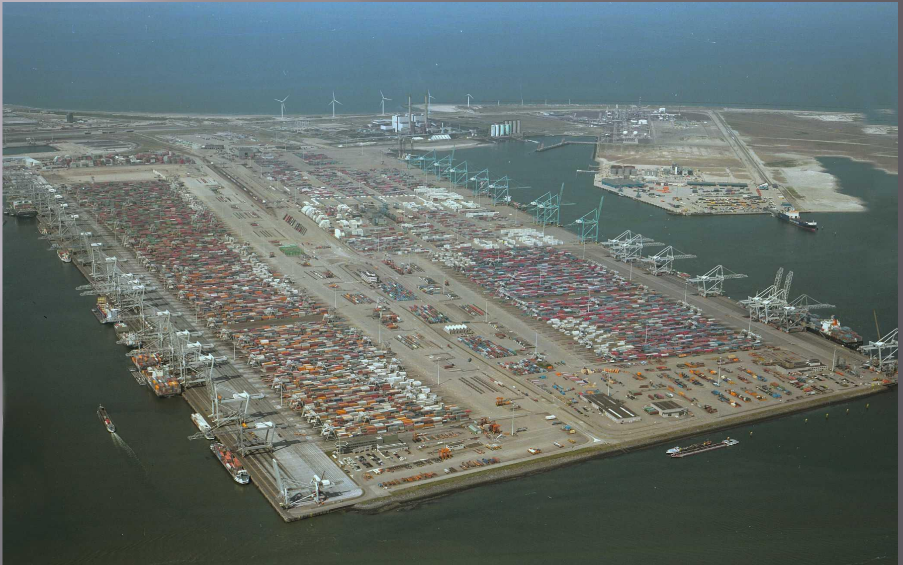
The general view at port
