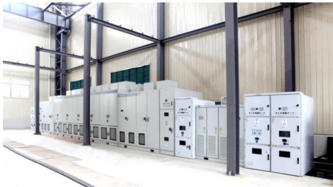
12 MW HV inverter for the first nuclear pump test station in Shanghai Apollo
