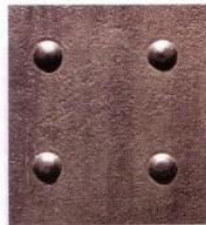
Solid rivets after installation
