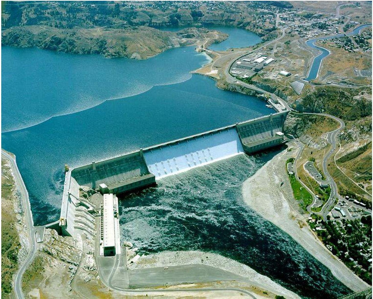
Grand Coulee Dam in Washington
