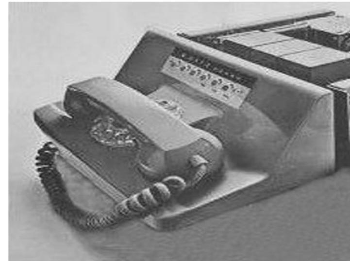
The first commercial modem Bell 103, operates at a speed of 300 baud.
