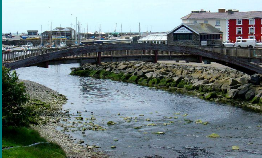
Footbridge over the Aeron
