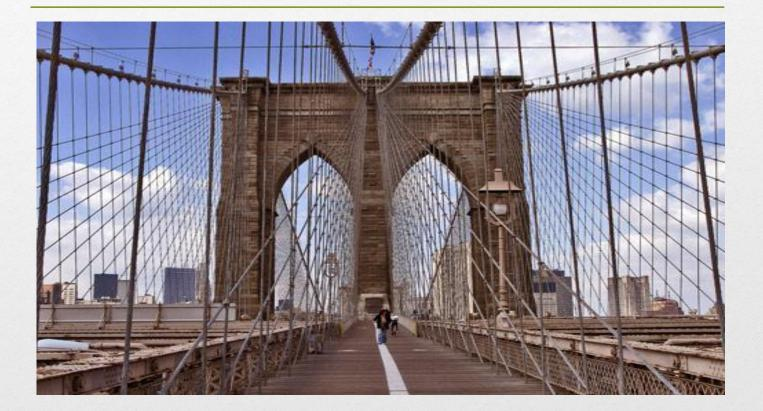
The Brooklyn Bridge was the first bridge to use steel cables and it held the record for being the longest suspension bridge for 20 years.
