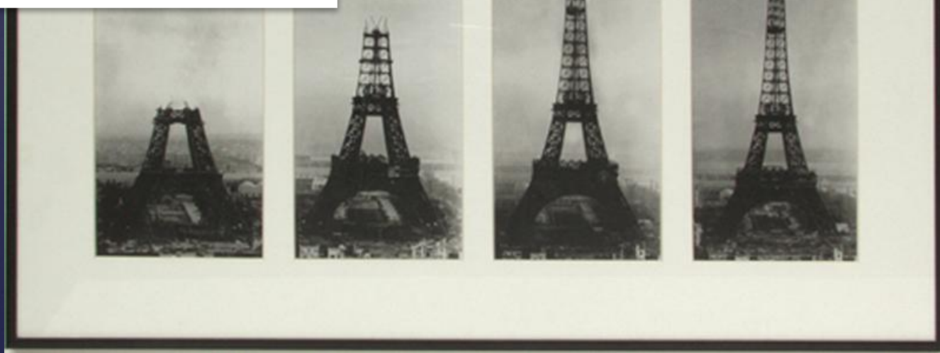
Building the tower in Paris on August 10, 1889
