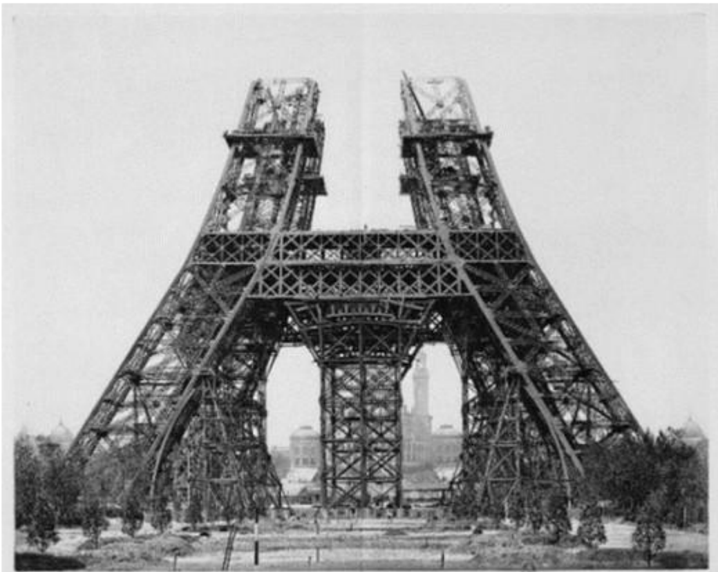
View of the scaffold
