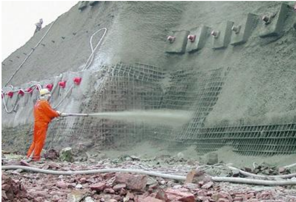
special spray gun V50 for shotcreting, max. 8mm grain size
