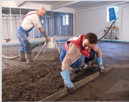
pumping of cement based floor screed (moist material)
