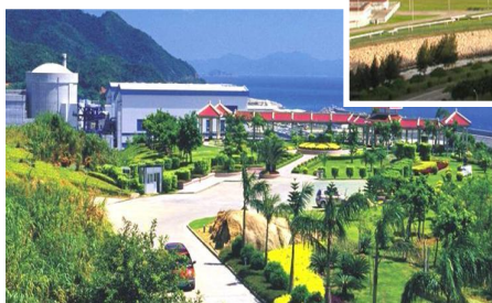
Ling'ao Nuclear Power Station Линаоская АЭС
