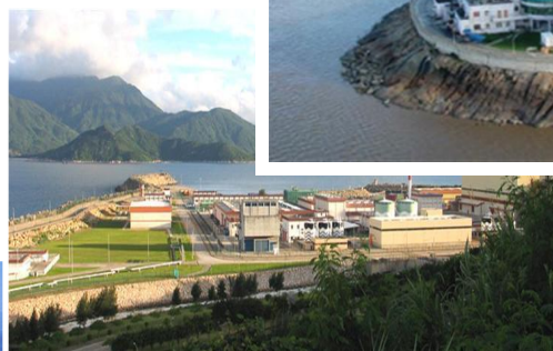
Daya Bay Nuclear Power Station Даяваньская АЭС
