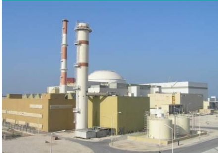
Iran, Buser NPP Unit 1 - 1000 MW
