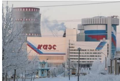
Russia, Kalinin NPP Unit 4 - 1000 MW
