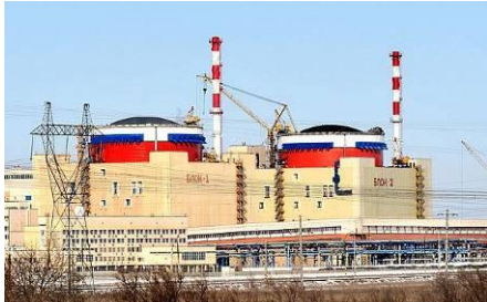
Russia, Rostov NPP Unit 2 - 1000 MW
