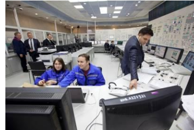
Russia, Rostov NPP Unit 3 - 1000 MW
