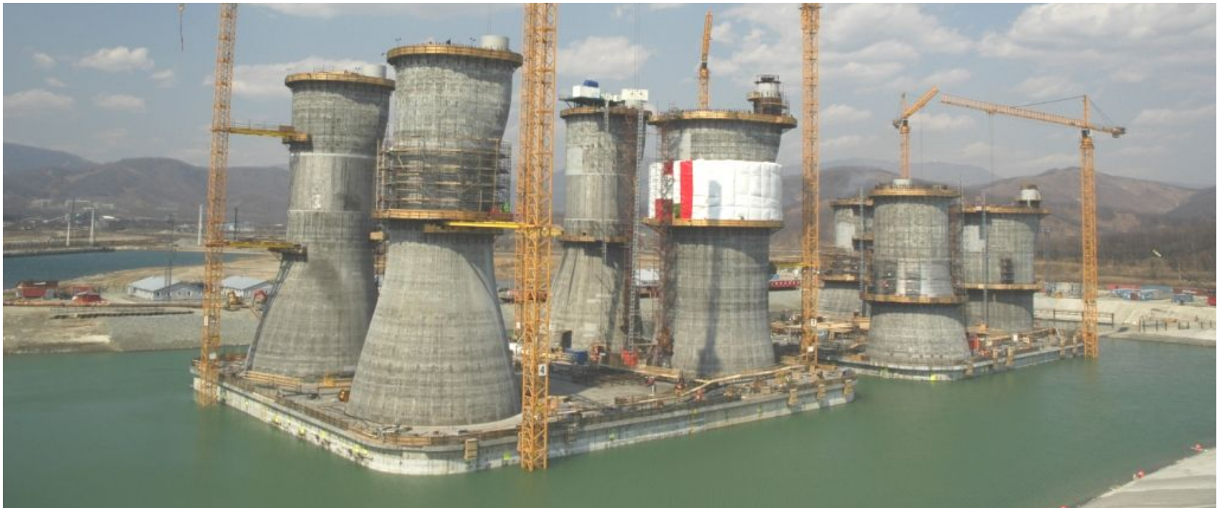
Concrete Gravity Base Structure Lun-A
