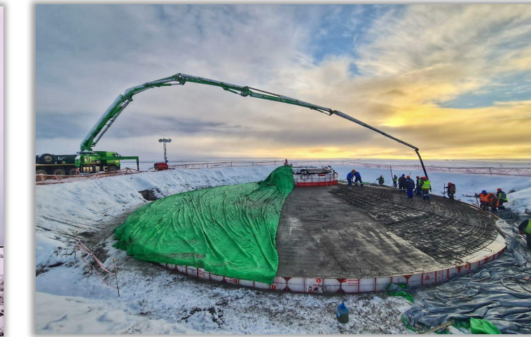
WTG FOUNDATIONS CONCRETE POURING
