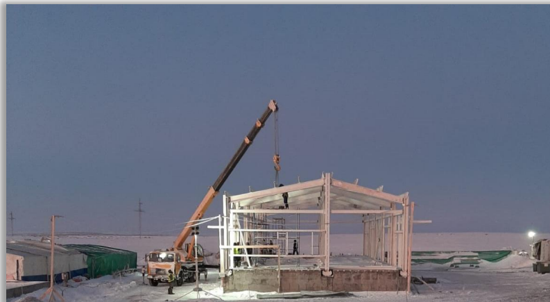
SUBSTATION – GIS 35KV – STEEL STRUCTURES INSTALLATION
