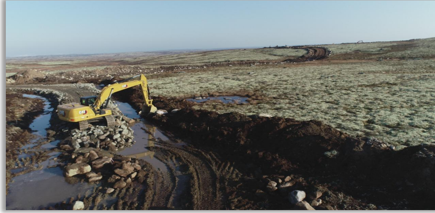
INTERNAL ROADS SWAMP FILLING AT SUMMER PERIOD
