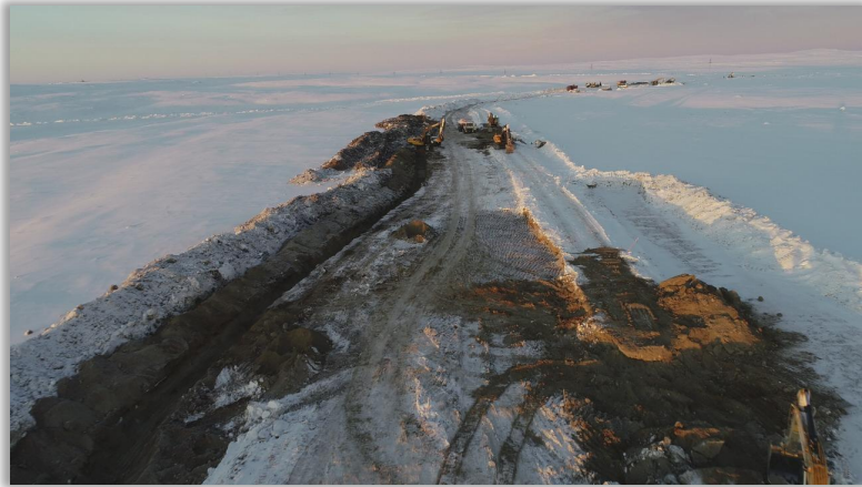
CRANE PADS EXCAVATION
