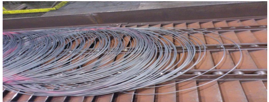
Laying bed "A"
