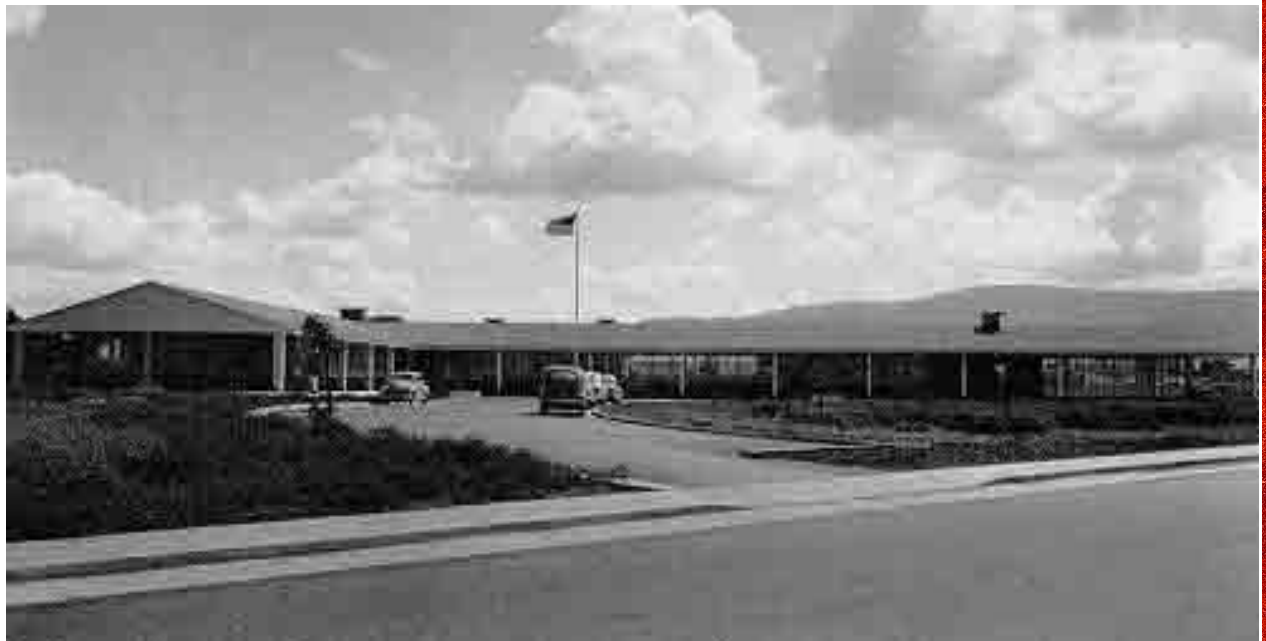
The First building of Silicon Valley First Varian Associates building, Stanford Industrial Park, Palo Alto, California, 1953.
