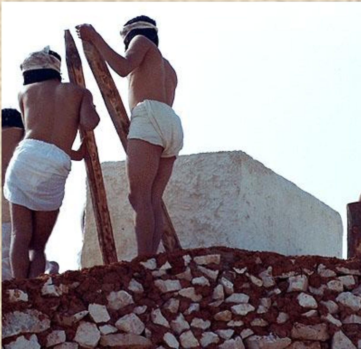
Rocking a block into position
