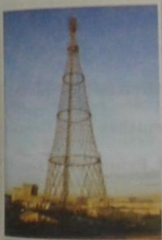
One of Shukhov's towers
