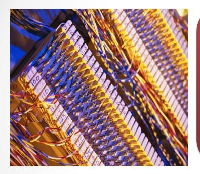
Older wiring closets sometimes have the same type of patch panels for both telephone and network support. These panels require punch-down blocks to make connections. Punch-down blocks are closely fit jaws that pierce individual wires to make a connection. They are somewhat difficult to use, and they also require specialized tools for connecting to the panel.
