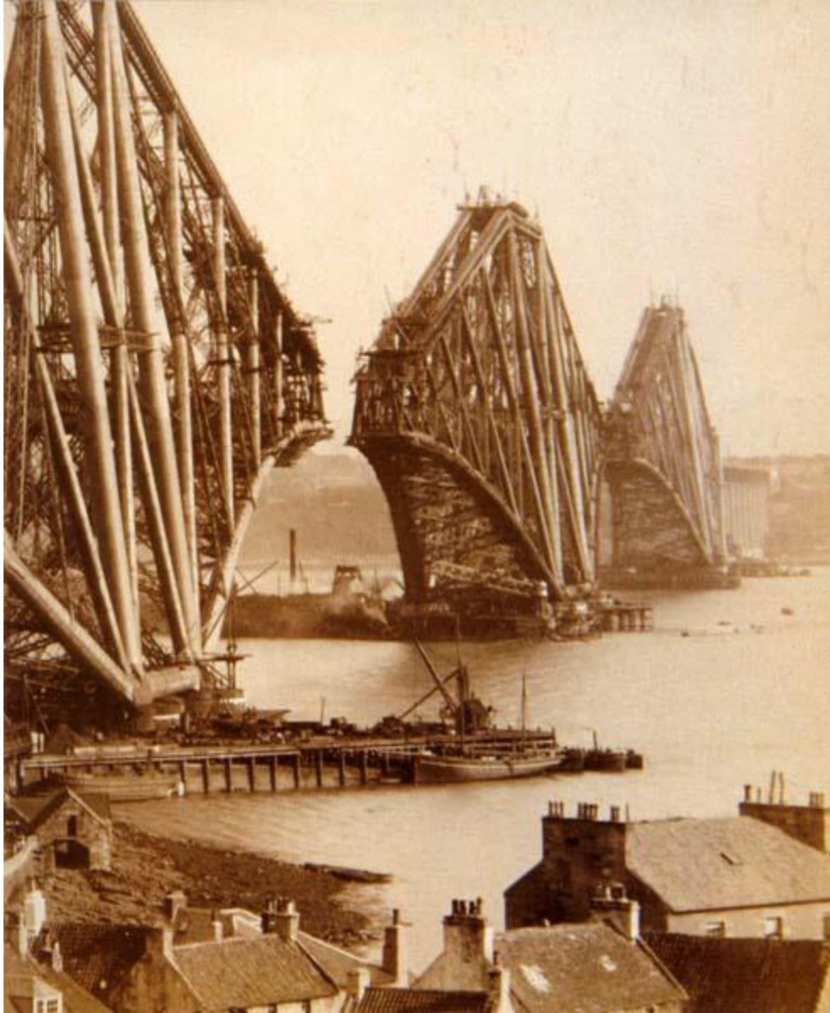
Forth Bridge under construction c 1888
