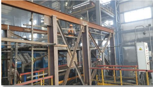
Middle conveyor support structure assembly
