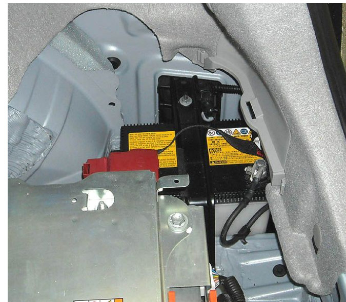
Auxiliary Battery (Sealed-type)
