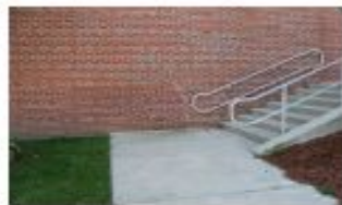
brick wall and stairs
