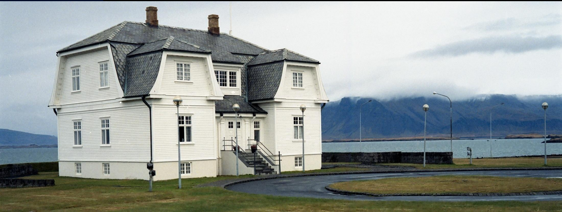
Hofde House, site of the Reykjavik Summit, October 11-12, 1986
