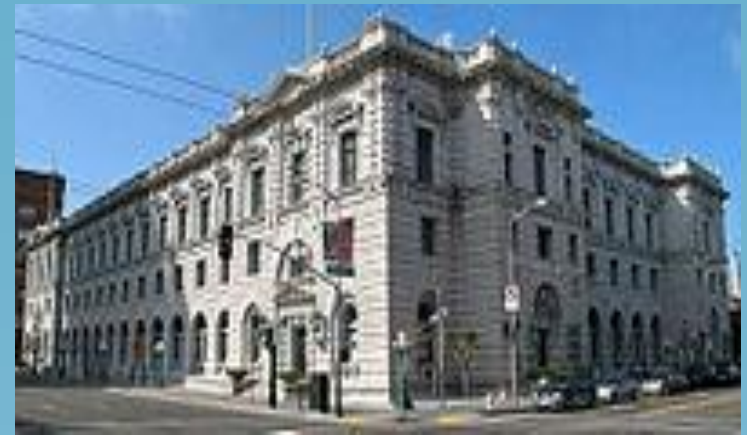
the building of the court of Appeals the James Browning in San Francisco
