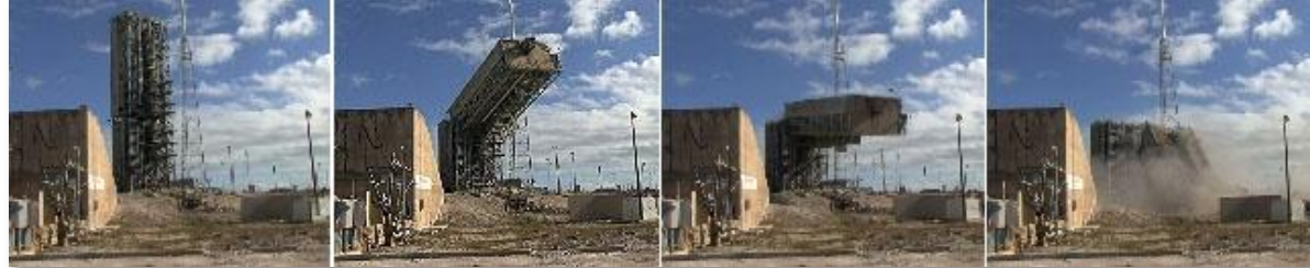
Demolition of legacy Umbilical Tower (8 January 2008)
