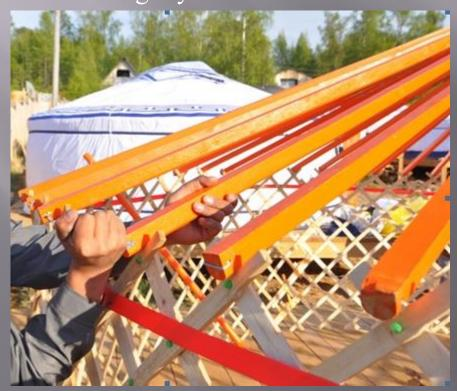
Toono is turned "upside down" and we tie struts stronger. We raise and put the tone on the stands in the center of the circle, orienting it from north to south, centering on the door.
