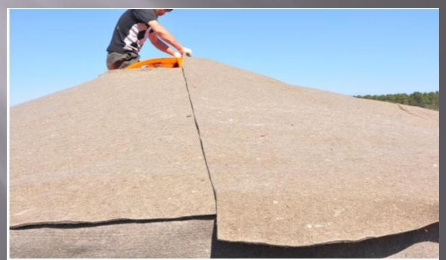
10. In the end we put on a cover, tightly tie it with ropes from the outside. We fix the erytho - the upper lid. For all the ends tie ropes - one end above the door will open and close, the rest will be permanently fixed, so they need to tie tightly.
