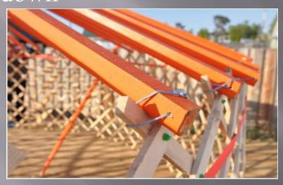
Unions are more convenient to insert outside the yurt. Fully install the union. Where necessary, there it is necessary to cut the ends of the union with an ax or chisel, so that the end of the union deep and densely enters the hole of the tono.
