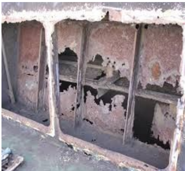
Inoperable fire damper. Wastage found after removing cover.
